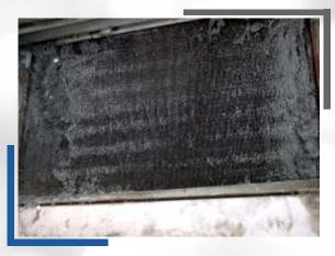
Allergic reactions are caused by dust particles, pollens etc. The AHUs usually have a provision for controlling the dust particles through various types of particulate filters. However these filters with large pore sizes are able to catch only the large dust particles, leaving the smaller ones circulating in the air.
